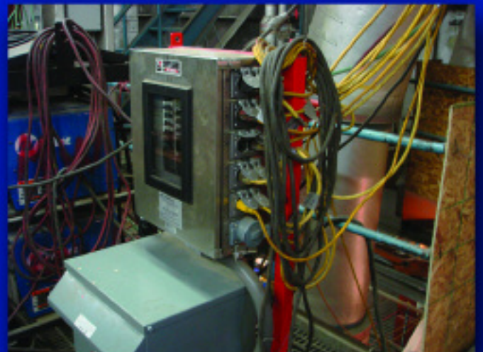
All 20 amp and 50 amp breakers are equipped with built-in G.F.C.I.'s
